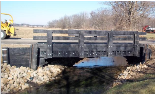
Bridge 174-0.56 over the Onion Ditch
